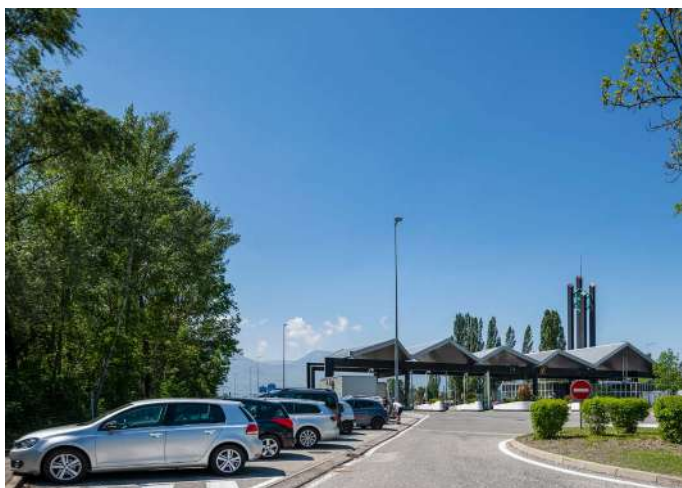
Parking relais péage autoroute Montmélian © Yannick Siegel
